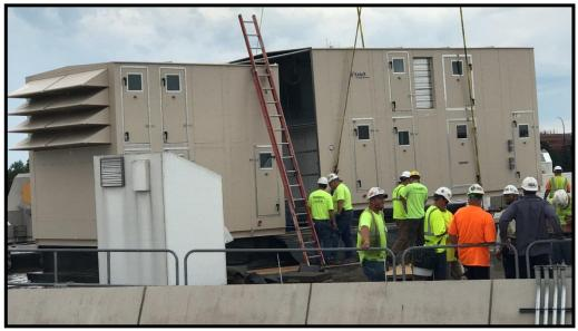
Featured Unit: Rooftop Sensible Flat Plate Energy Recovery Ventilator with Chilled Water and Hot Water Coils
