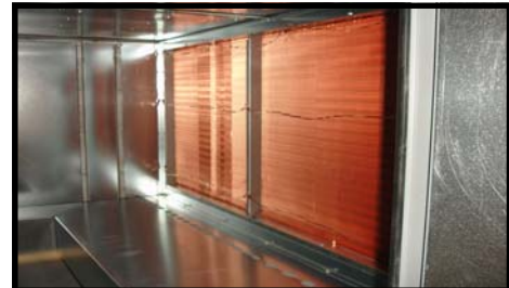
The EA Blower and All-Copper HW Coil
