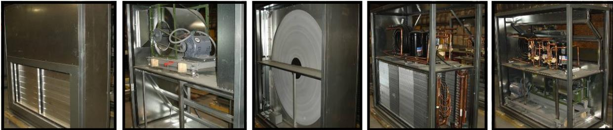
From left: The end section contains the OA damper; the next section contains the exhaust blower (top) and OA filter rack (bottom); the middle section houses the heat wheel; the next section contains the DX and Hot Gas Reheat coils (bottom) and two compressors (top); and the last section houses the twin supply blowers (bottom) and another two compressors (top).
